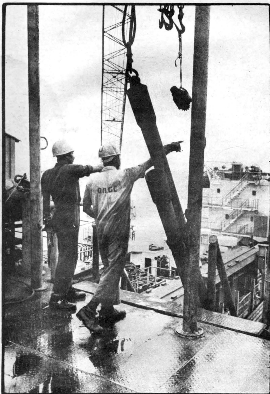
ON THE RIG FLOOR: Jobmen direct the descent of the heavy sharp-edged drilling bit.
