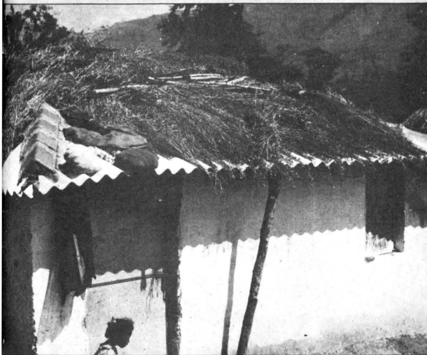
Weighting down an asbestos roof with tiles and thatch.
